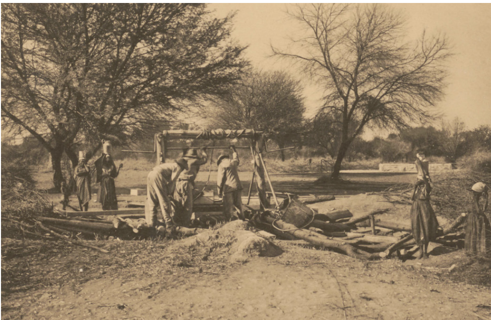
Fig. 3: image titled „Otavi-Bahn: well construction at Otjivarongo, km 378.“
